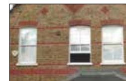
Timber windows set behind a brick reveal
