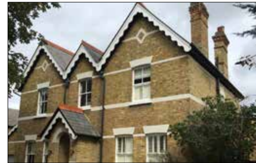
Gables with decorative barge boards and decorative brick work
