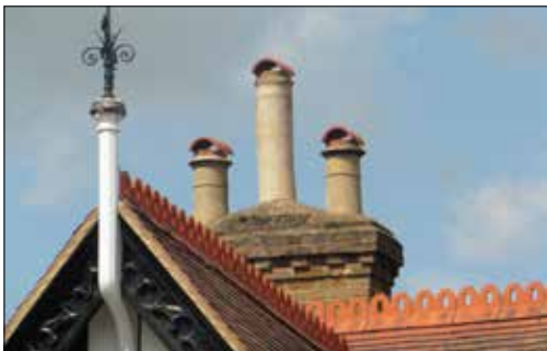
Example of decorative ridge tiles and barge boards, combined finial and kingpost, and unique chimney design
