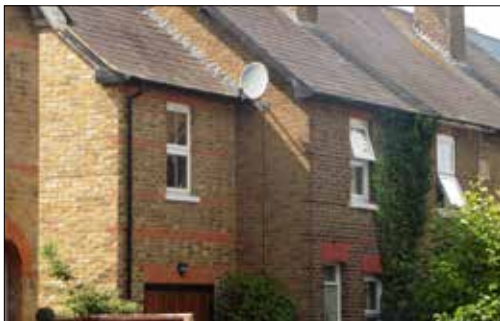
Brickwork banding carried through from original home onto a well proportioned extension (size compared to original and windows)
