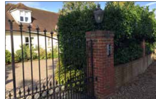
Coordination between railings and gate, and gateposts and wall pillars.
