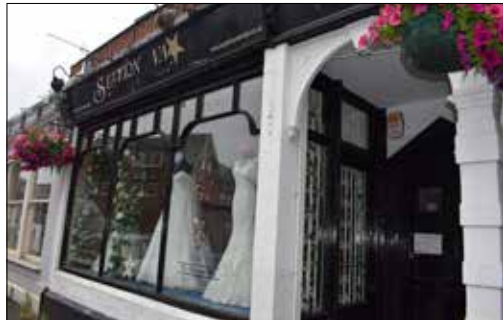
Simple and elegant sign writing and window lettering, appropriate fascia lighting, decorative internal security grills
