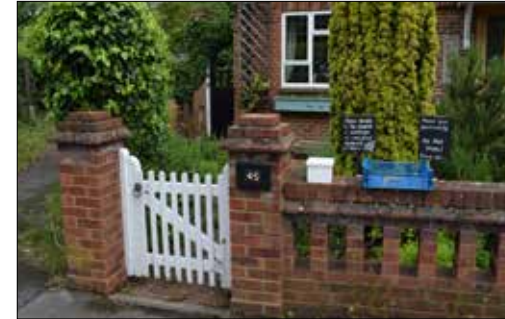
Decorative wall, with proportionate gateposts and traditional gate design
