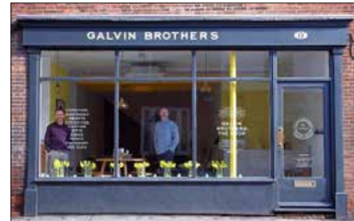
Contemporary shop front design with traditional proportions and detailing, simple signwriting including window lettering.
