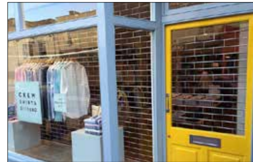
Example of internal security grilles which provide security whilst providing visual interest and lighting to the street.
