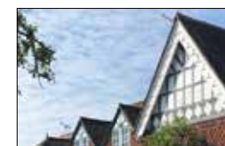
Decorative timber boarding on gables
