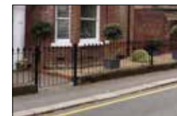
Metal work details
