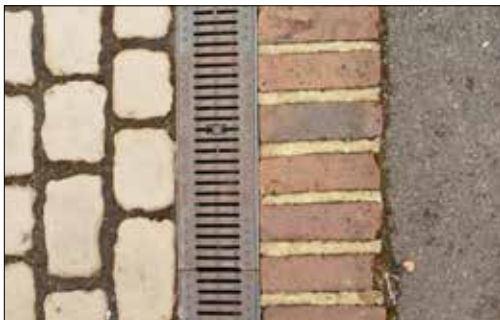
Utilising red brick to match walling next to the curb, and parallel placement of the grate reduces its visual impact
