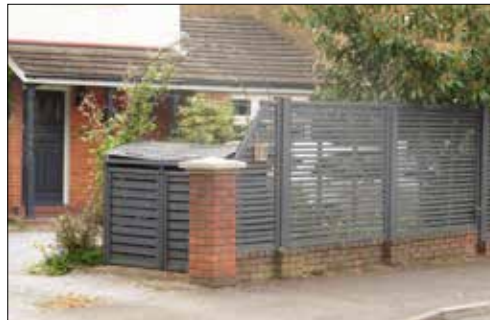
Example of integrated bin storage and fencing, including planting to further soften the design
