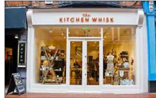
Contemporary shop front design with traditional proportions and detailing, extruded lettering and use of accent colour.
