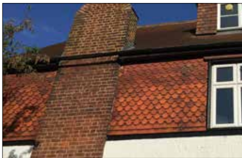
Example of a combination of fish-scale hanging tile in terracotta at first floor level
