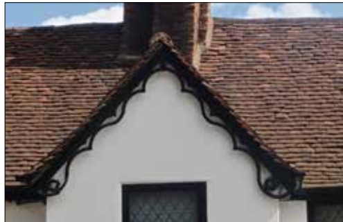
Decorative barge boards on gable ends
