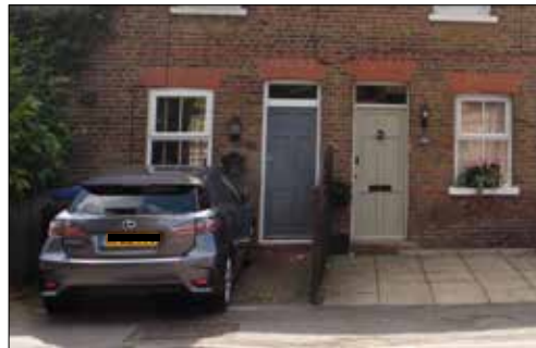
Example of retaining dividing railings between driveways when removal of frontage boundaries is necessary to provide parking
