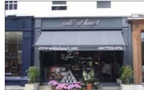
Use of muted contemporary colour, extruded fascia lettering, and provision of an integrated sun awning
