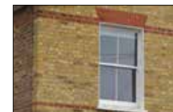
Contrasting brick banding details (buff and red brick)
