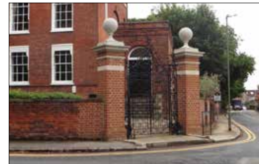
Corner gate detailing on river frontage and blind boxes on windows
