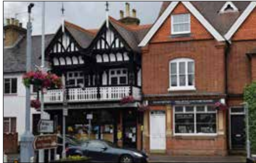
Holistic frontage design, including traditional proportions and detailing, with signwriting and window design
