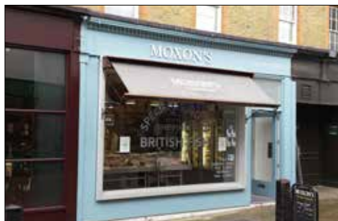
Integrated sun awnings allowing continued visibility of the fascia, contemporary signwriting on window and simple use of colour.
