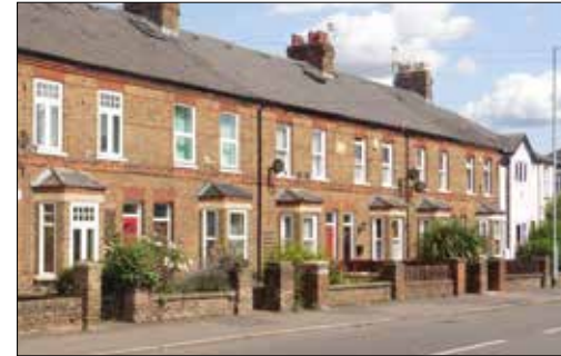
Terraced with small front gardens with boundaries retained. Slate roofs including dormer windows
