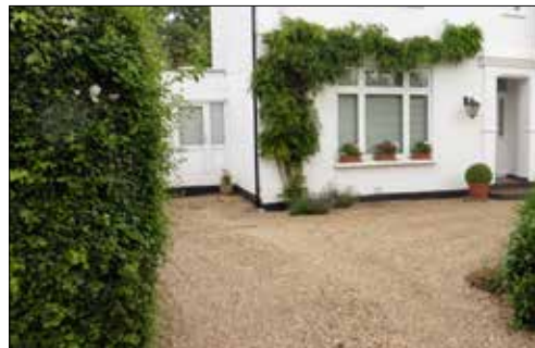
Example of gravel as a permeable surface treatment where complete coverage is required, which can also be planted through
