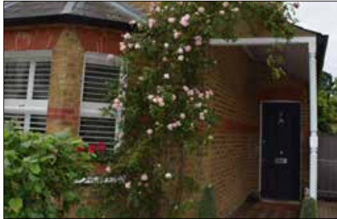
Distinctive side porches and entrances
