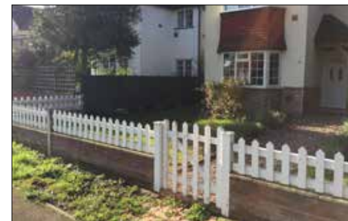
Combination of a simple low wall and fencing with a coordinated gate and gateposts allow views of the garden beyond.
