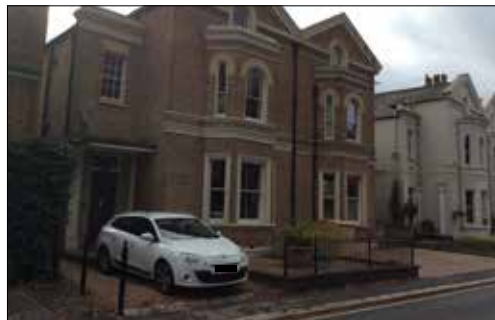
Stone detailing, and double-height bay windows on High Street
