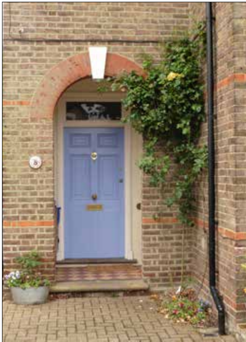
Example of an inset porch offering shelter, exterior storage and incorporating climbing planting without the loss of paved area
