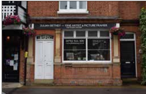
Reuse of a former bank - contemporary signwriting, window lettering for additional detail, and internal security shutters
