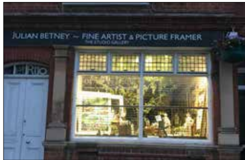
Internal lighting of the window display.
