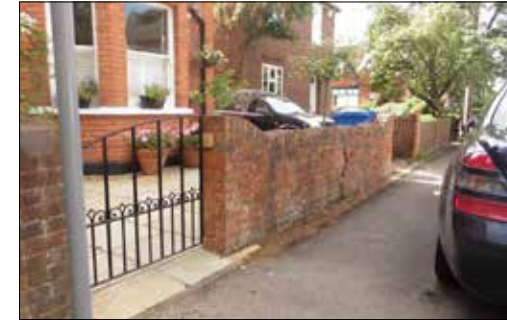
Example of separate pedestrian and vehicular gated access, with wall retained, providing parking and boundary definition
