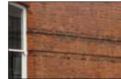
Extruded banded brick work and red brick (Flemish Bond)
