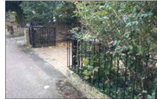
Decorative metal railings on low brick walls with associated gates
