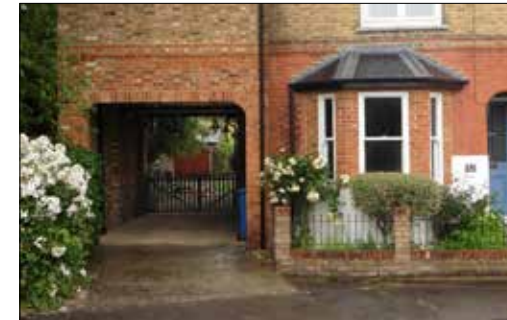
Example of a side extension which includes an undercroft for parking and access to the rear of the property
