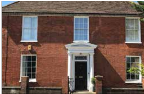
Example of replacement wooden sash windows with inset fitting
