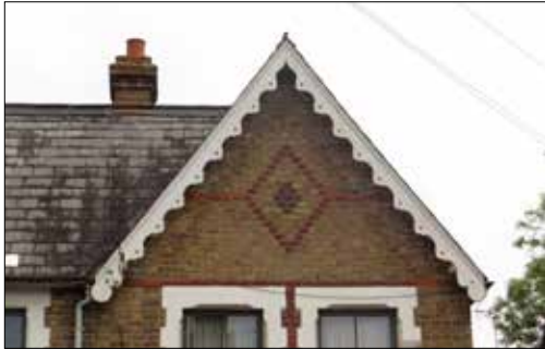
Gable ends - including decorative barge boards and decorative brick work
